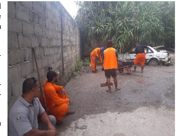
Inmates cleaning mud outside the old correctional centre after weeks of rain
